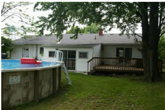
Decking and above ground pool
